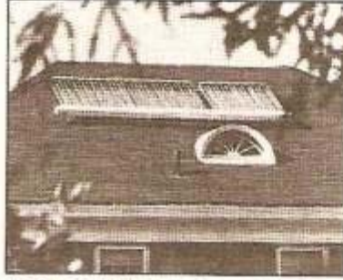
HOME COMFORT: Twenty-four glass bulbs on the roof of this home in upstate New York provide all the family's hot water (80 gallons a day). The total cost of installation was $2,500.
